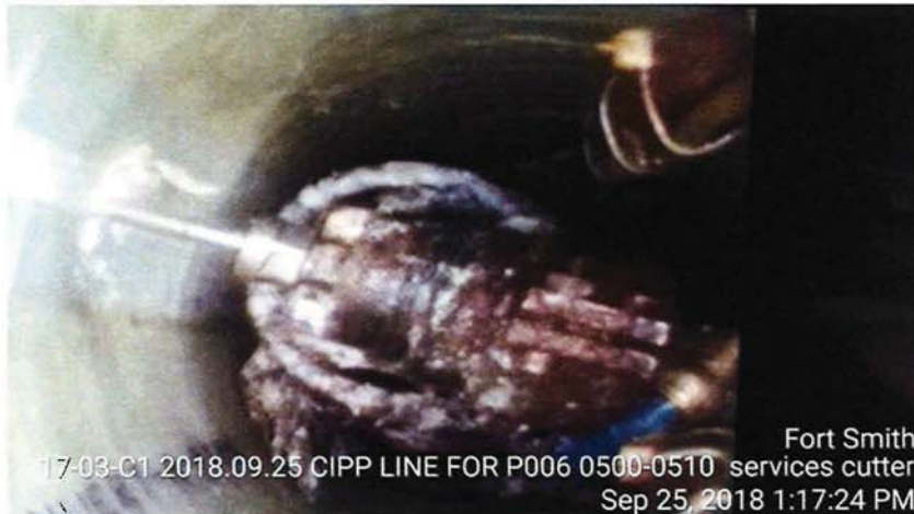
Robotic Cutter Reinstating Service Connection
