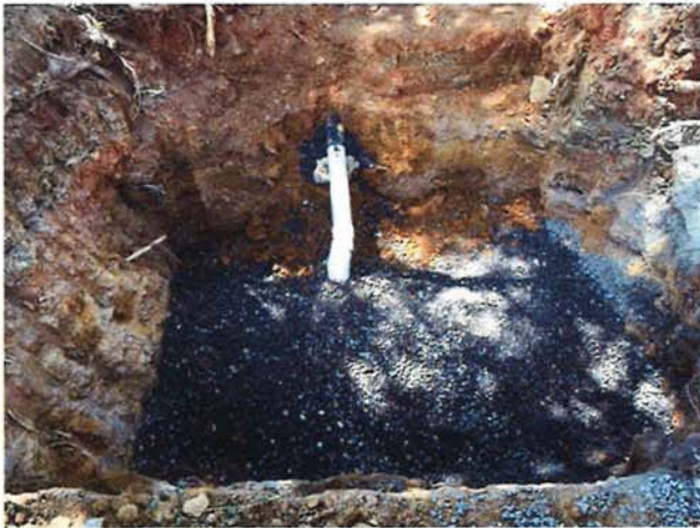
Lateral Line Repair
