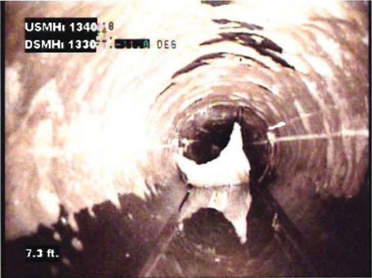
Spalling Pipe Wall & Hanging Gasket
