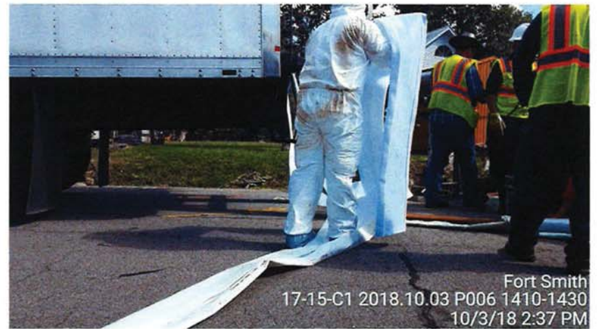
Felt Liner Tube Insertion
