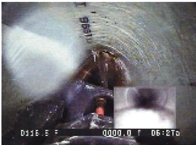
I&I At Service Line Connection
