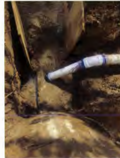
Service Line To Main Inserta Tee Connection
