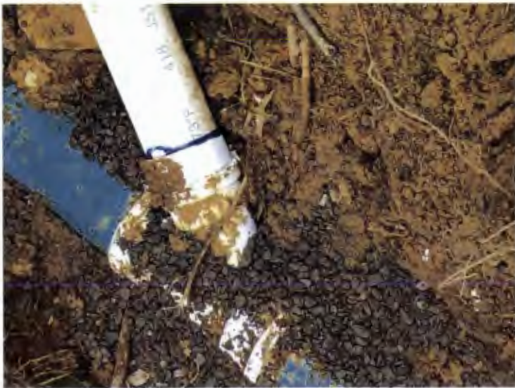
Service Line To Main Wye Connection
