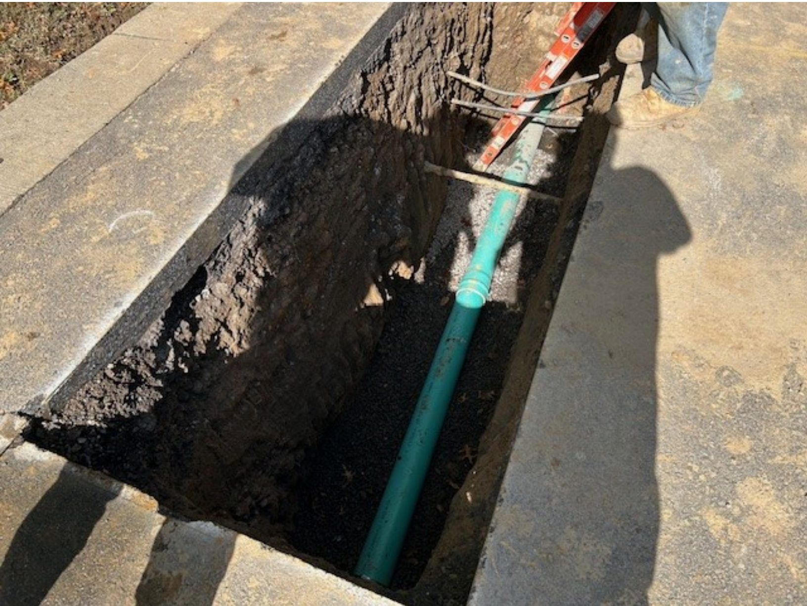
(Site A) 8-inch PVC pipe "point repair."
