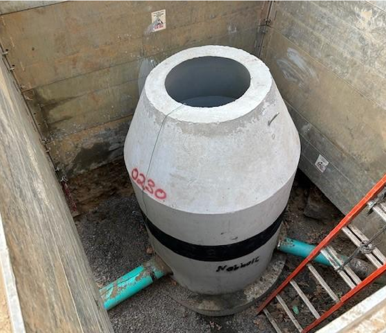
(Site B) New "pre-cast" manhole with new connections.
