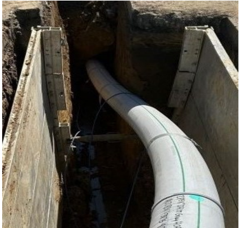
REPLACEMENT OF SANITARY SEWER MAIN LINE USING PIPE BURSTING METHOD
