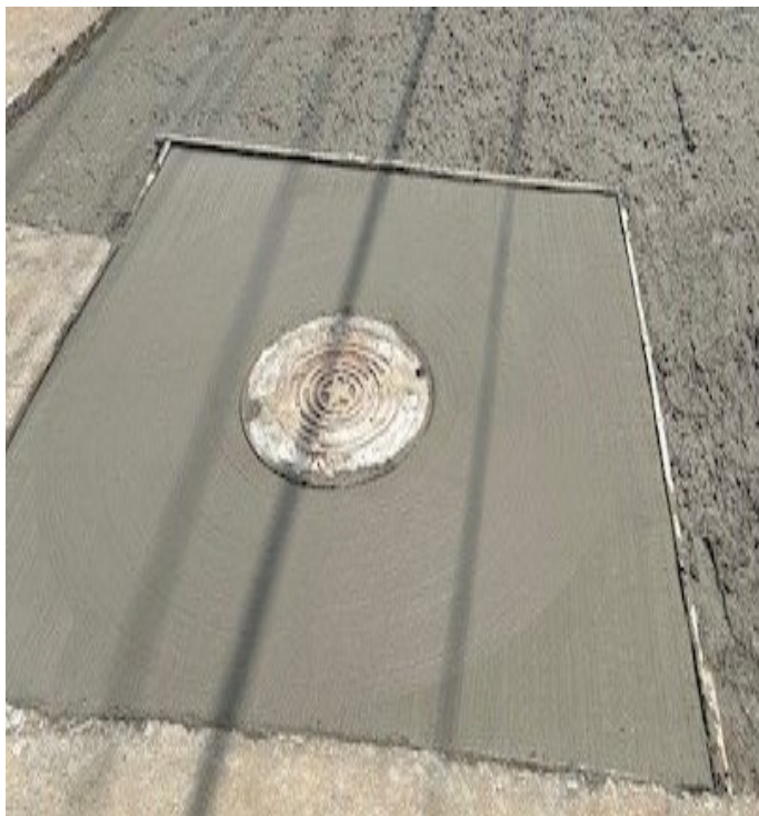
SITE RESTORATION PROCESS AFTER REPLACEMENT/REHABILITATION OF SANITARY SEWER SYSTEM
