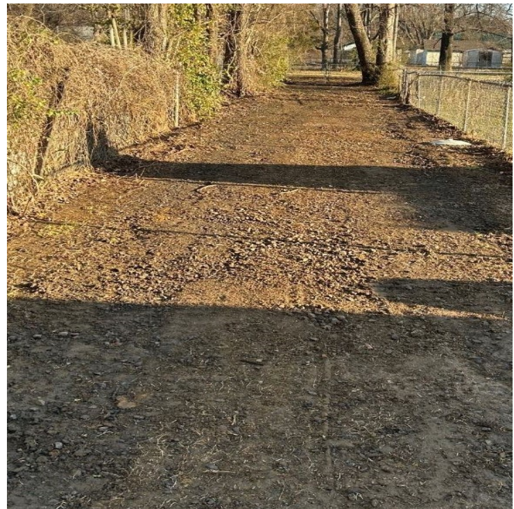
POST-REPAIR SITE RESTORATION FOR SANITARY SEWER MAIN LINES
