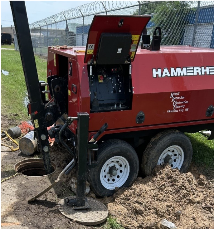
REPLACEMENT OF SANITARY SEWER MAIN LINE USING PIPE BURSTING METHOD
