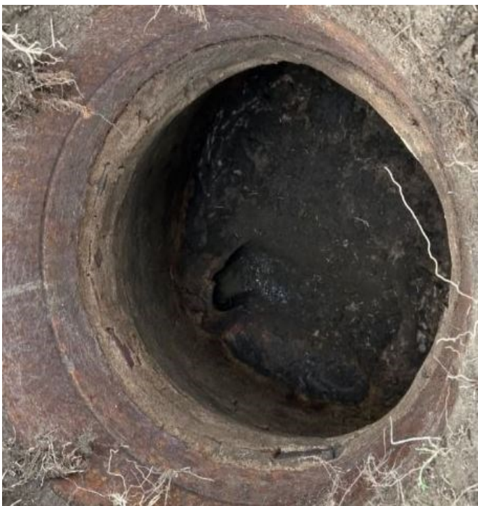
EXISTING MANHOLE CONDITION BEFORE REHAB OR REPLACEMENT WORK
