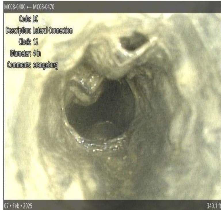
PRE-CCTV VIDEO INSPECTION OF SANITARY SEWER LATERAL CONNECTION
